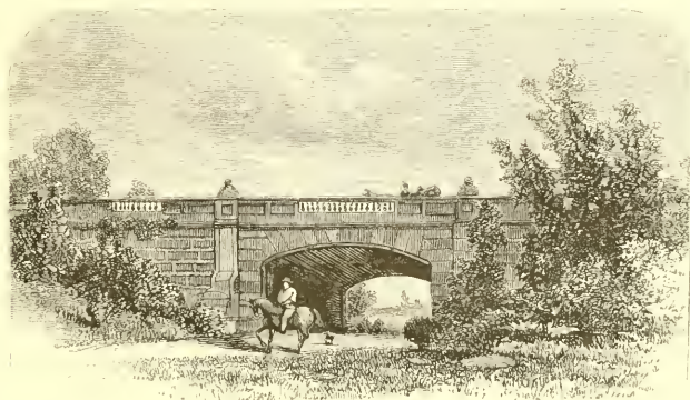
BRIDGE OVER THE BRIDLE PATH NEAR ARSENAL.
